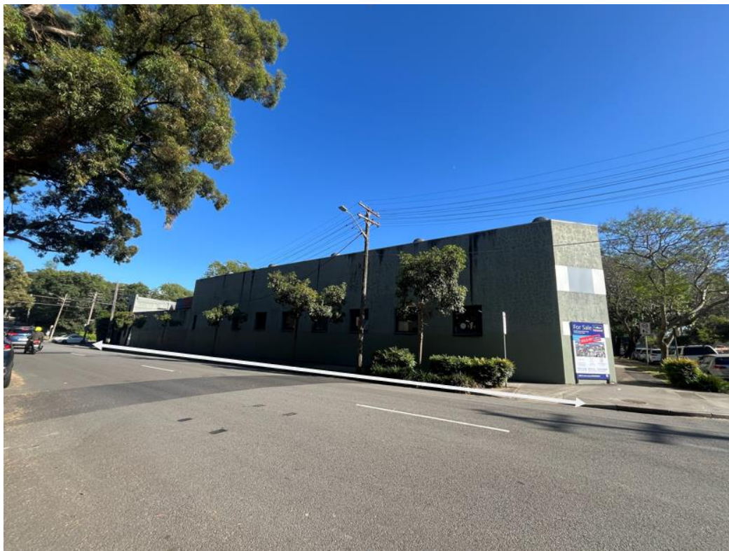
Figure 2: Site viewed from McEvoy Street
