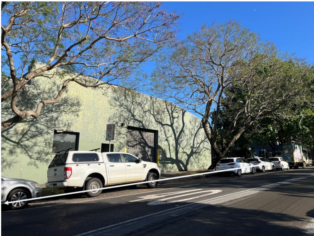
Figure 4: Site viewed from Young Street
